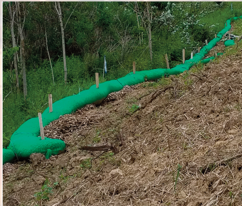
Top photo: Undergraduate research assistant Zackery Whisler working in ArcMap on well pad project Bottom: Example of silt sock use on-site
